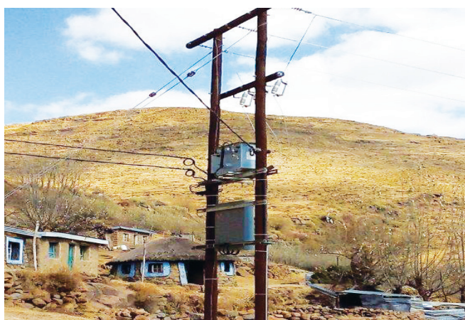
Koporale electrification Project in the Phase 1B
