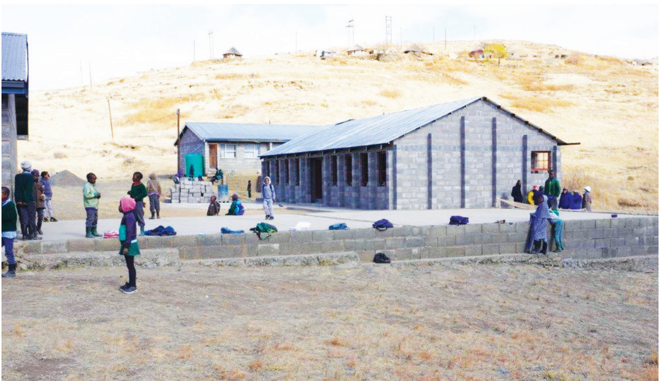
The two classrooms being constructed at Montsi Primary School
