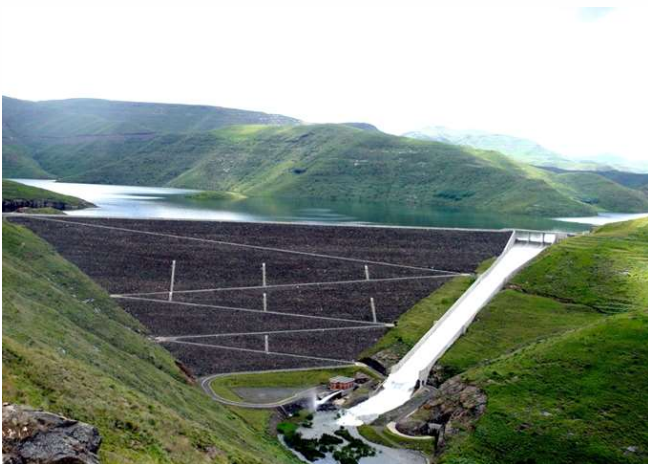
Figure 6: Mohale Dam spilling in April 2011
