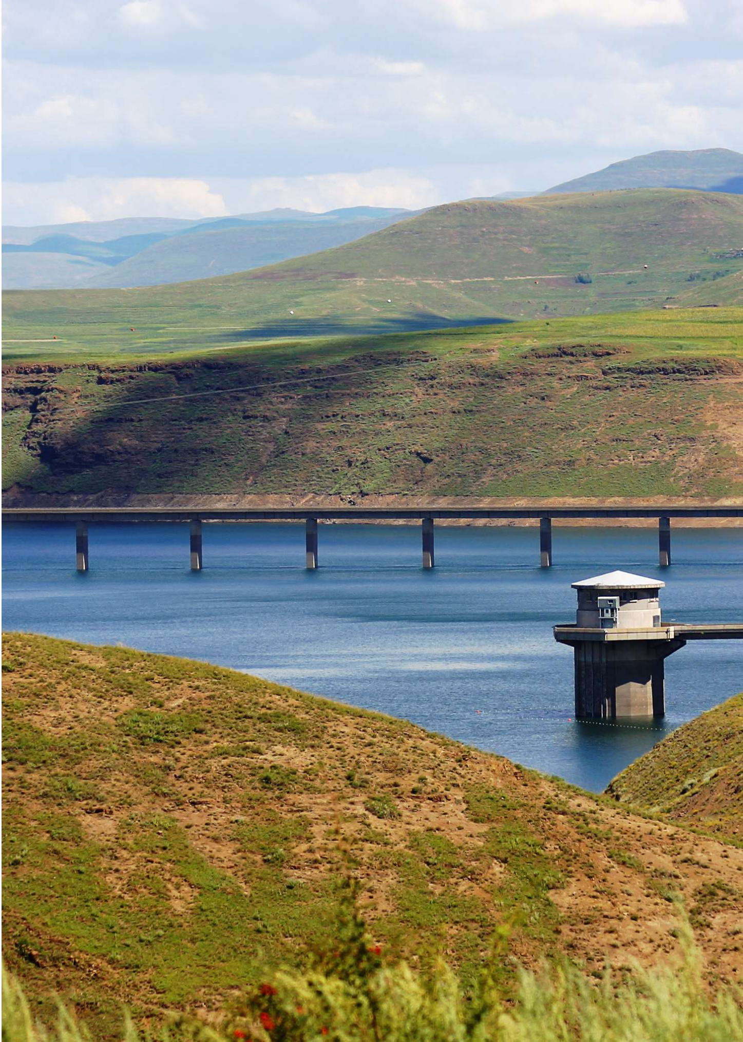
Maliba-Mats'ó Bridge and Katse Intake Tower
