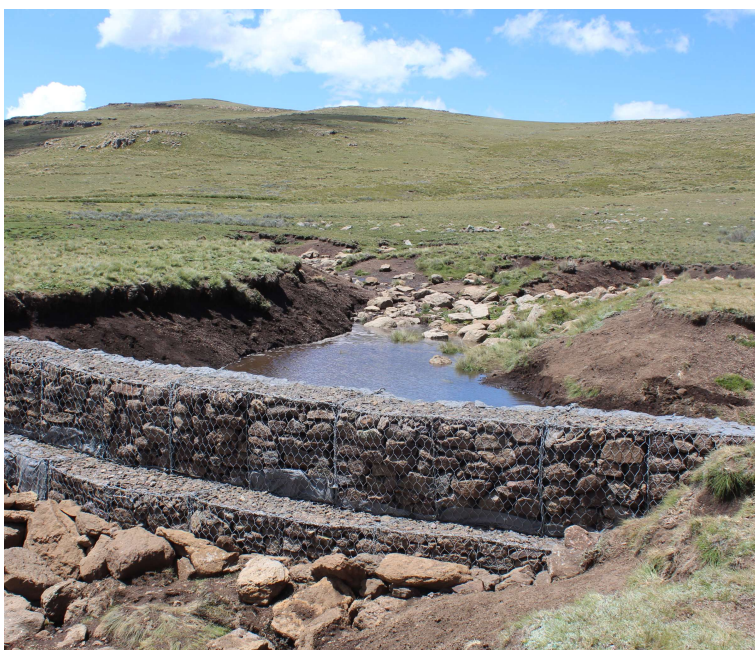
Brush control and gabion construction at Malingoaneng rangeland and Motseremeli wetland
