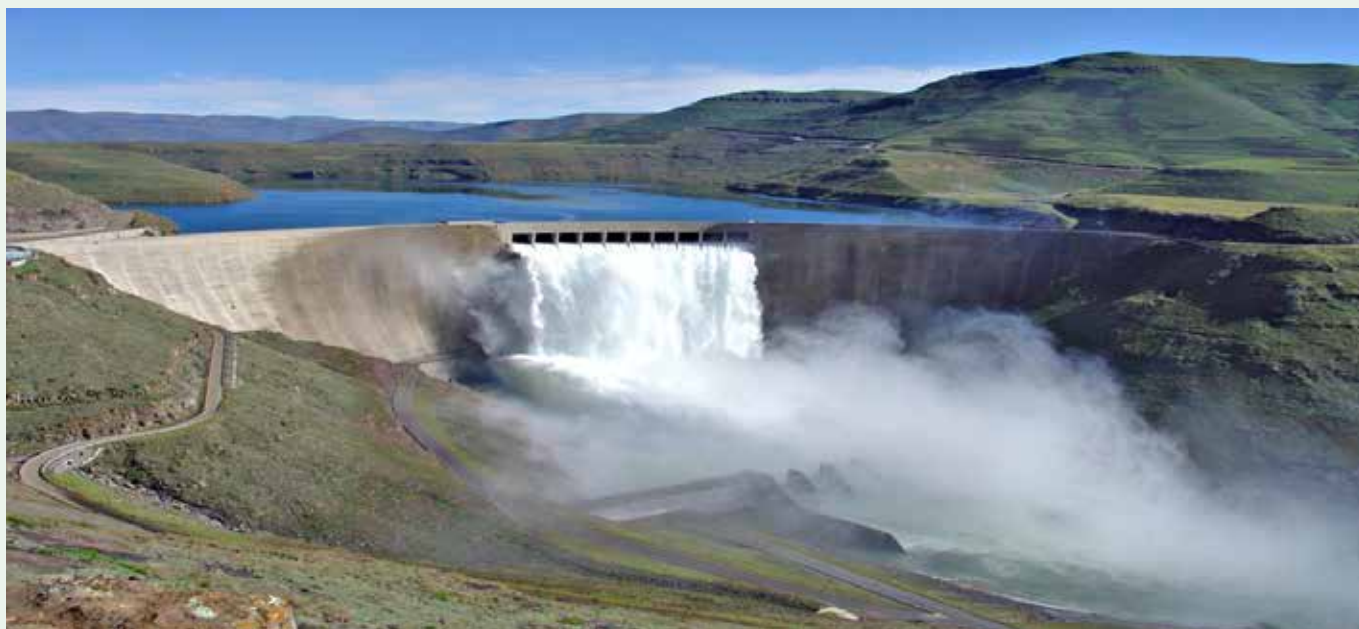
The Katse Dam spilling
