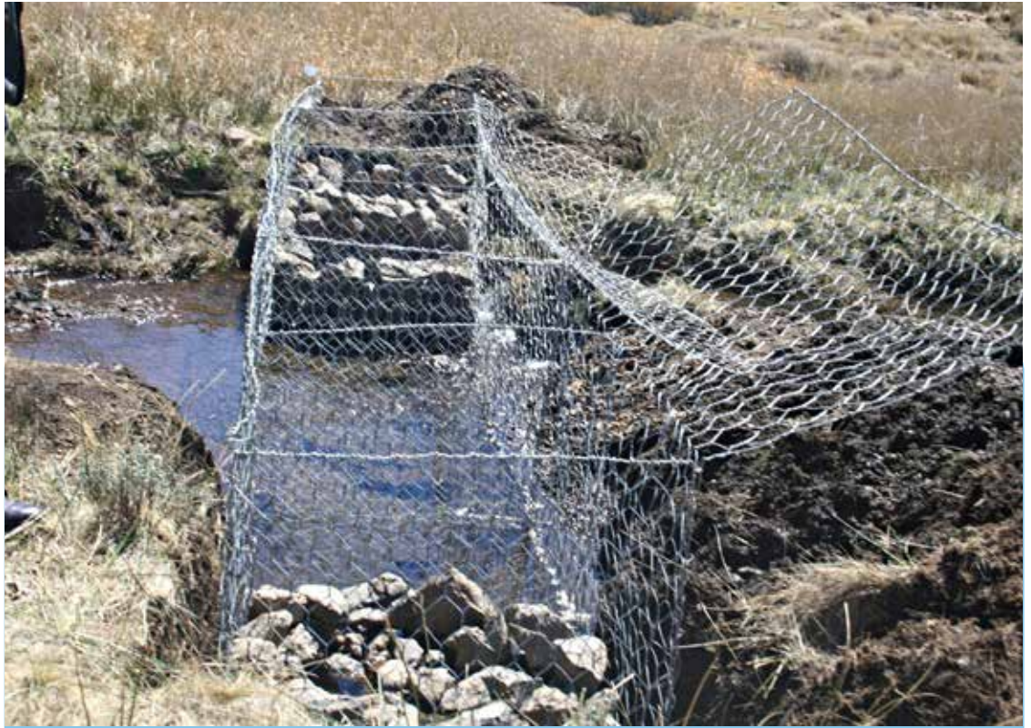
Land rehabilitation through gabion construction
