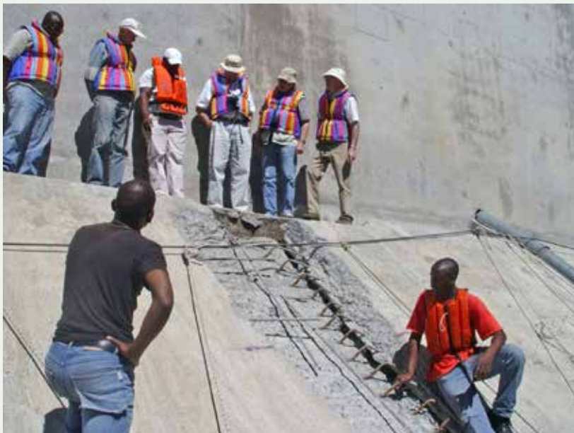
On-going repair works on the Mohale Dam face slab
