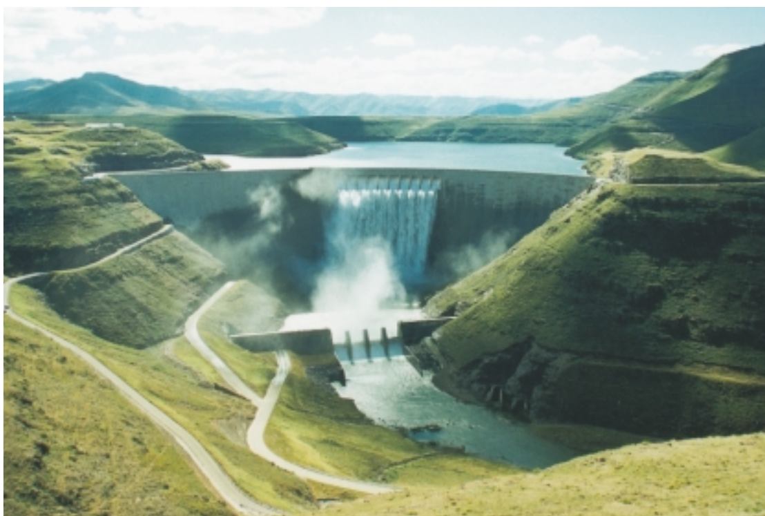
Katse Dam – the main storage of water for the Katse Reservoir could play a vital role in the fisheries in the development project.
