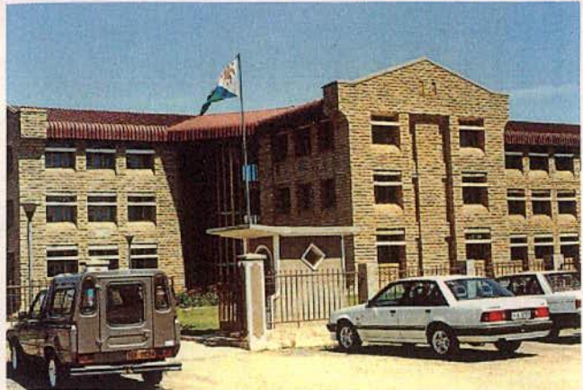
Phase I Government Office Complex – Qhobosheane in Maseru. Sample of work done by Kopanang Steel Fixers
